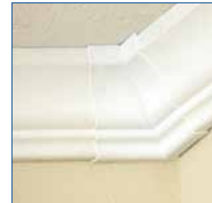
Left and right copes come together to form a perfect inside corner
